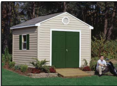
Figure 1 - Typical vinyl-sided shed with gable-style, composite shingle roof (Example only)
